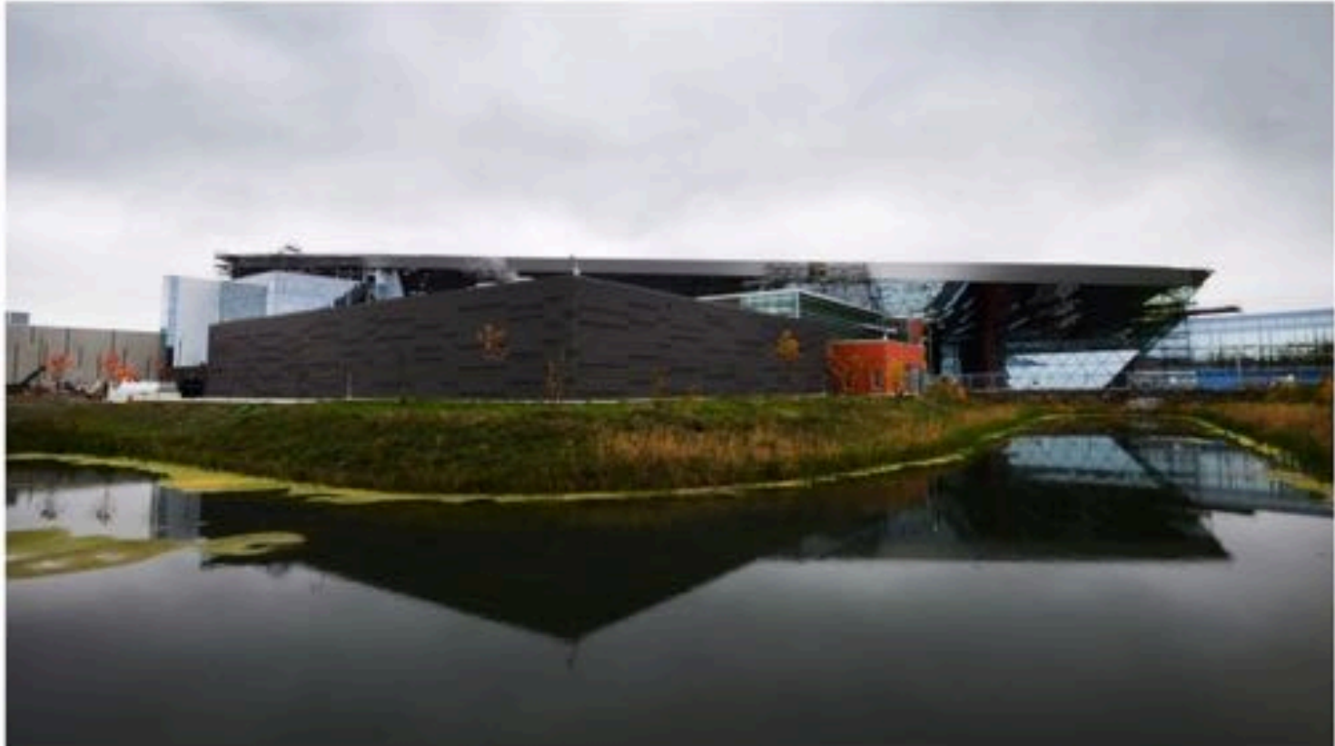
The new Communications Security Establishment Canada (CSEC) complex is pictured in Ottawa on October 15, 2013. (Sean Kilpatrick / THE CANADIAN PRESS)
